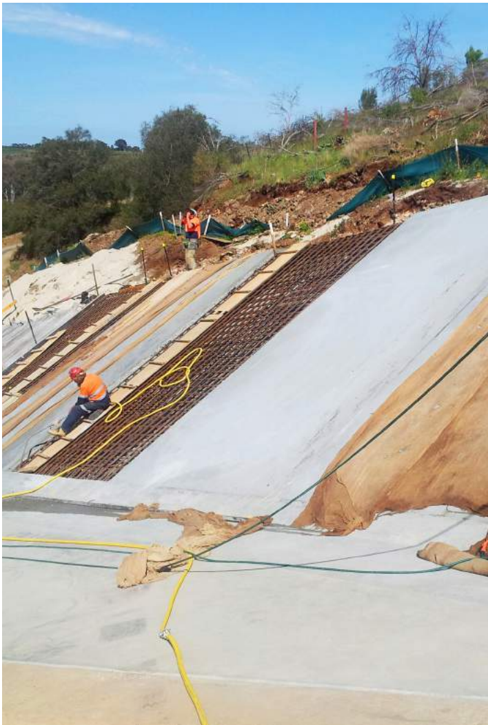
♦ Roller screed used on slopes
