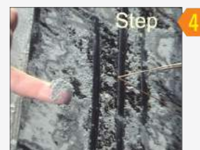
Hard concrete is turned into paste to be easily removed.
