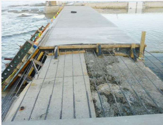
♦ FRP rebar used in iconic Merewether Ocean Baths upgrade
